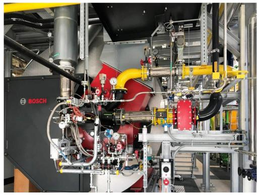
A Bosch steam boiler equipped with a multi-fuel firing unit for using hydrogen, natural gas and light fuel oil.
